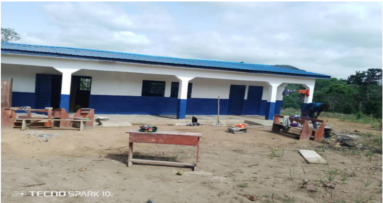
Entire classrooms floor concretes redone
